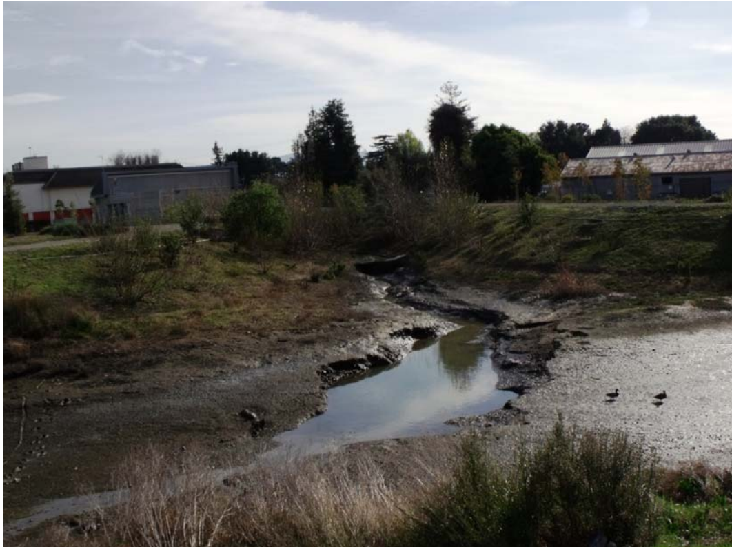
Figure 1 - Photograph of Vertical Drop Structure Downstream of Palo Alto Pumping Plant
